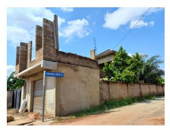
Because they lack trees in any great quantity here, buildings are made of cement and concrete products. Concrete blocks are often made by hand and are not as durable as the machine made ones so a finish coat is added as a protectant. When the project takes far longer than anticipated, the results can be startling when it becomes evident the mortar around the bricks is stronger
