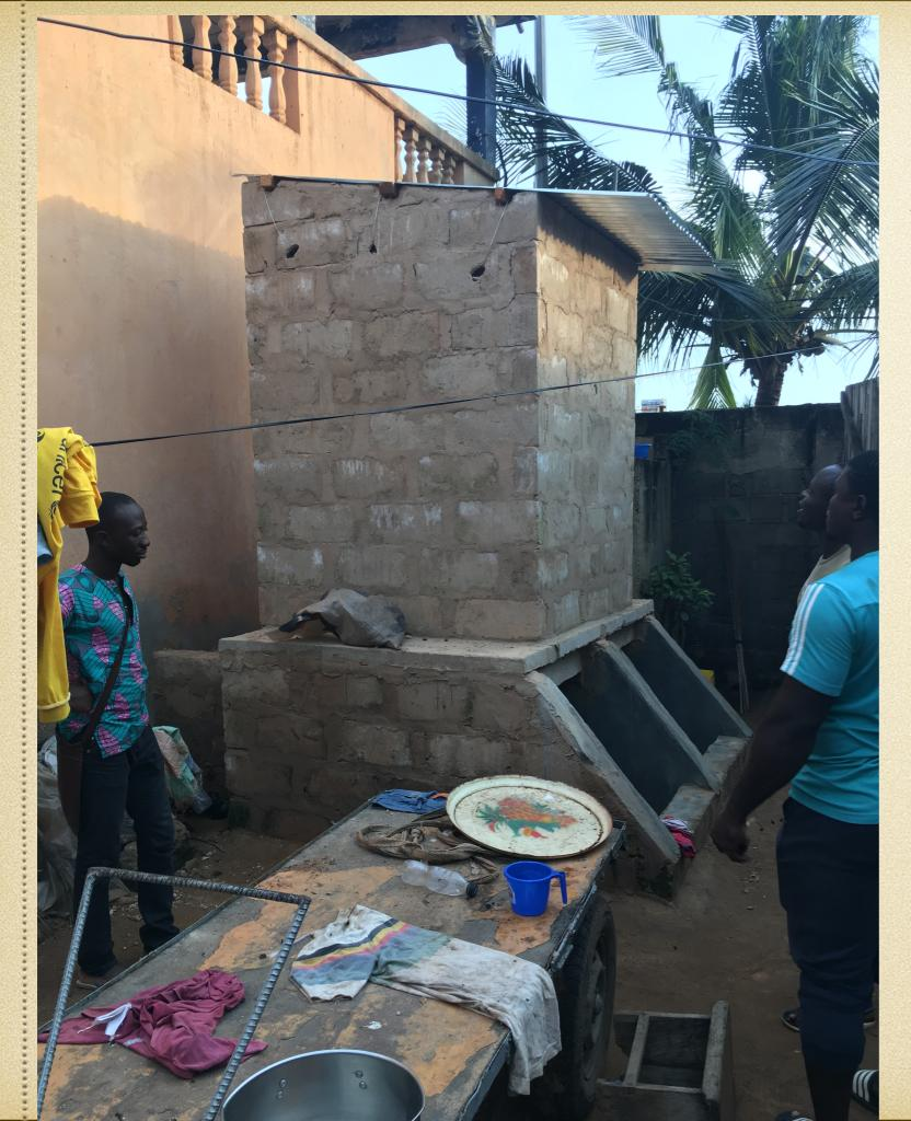
You can see the holes in the cement blocks and the wires wrapped around the boards that the roof is nailed to.
