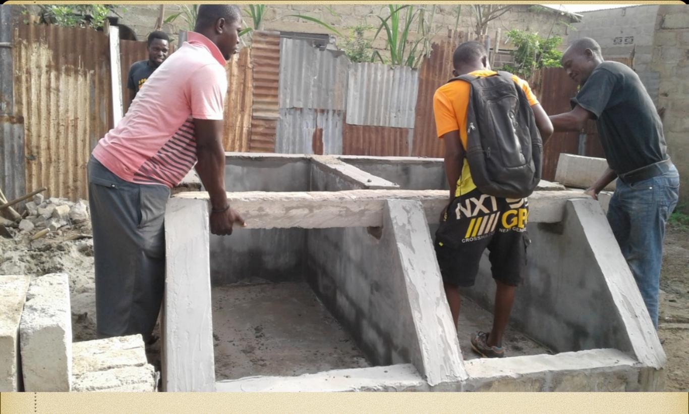
This rebar reinforced beam will provide needed support for the concrete floor and privacy cabinet.
