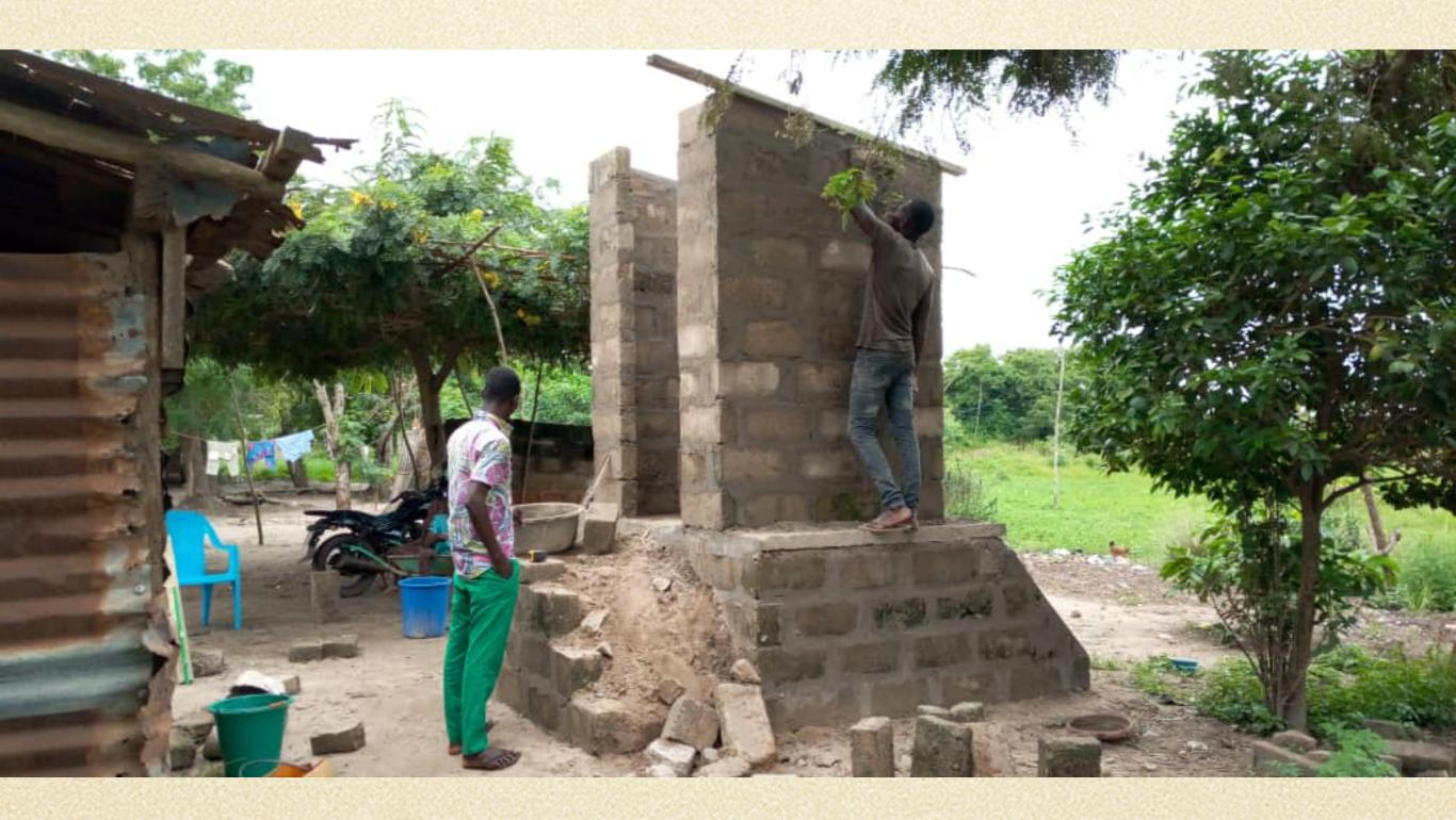
The bricklayer must make sure the angle for the roof is accurate. He makes small holes in the bricks so the roof can be tied in place by wires.
