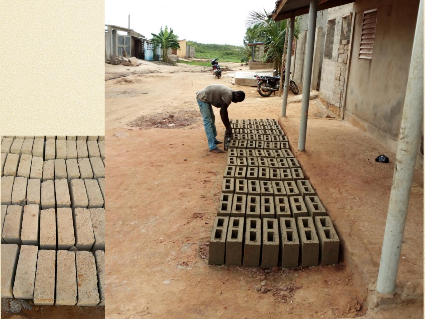
The bricklayer sets up the two chambered base for the Dignity Toilet making sure that the back end will stay in the direct sun.
