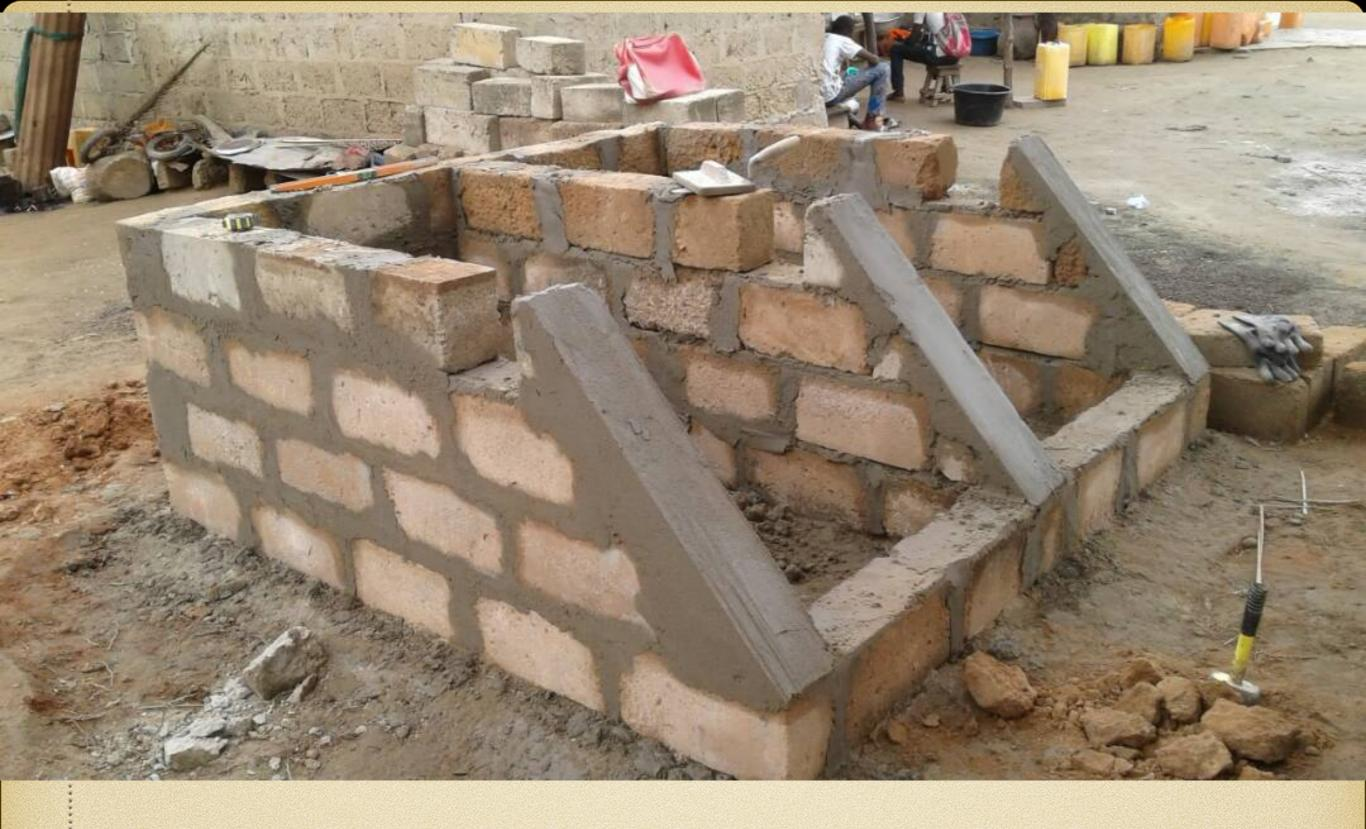
The rear of the Dignity Toilet base is notched to hold a cement beam that will support the cabinet floor.
