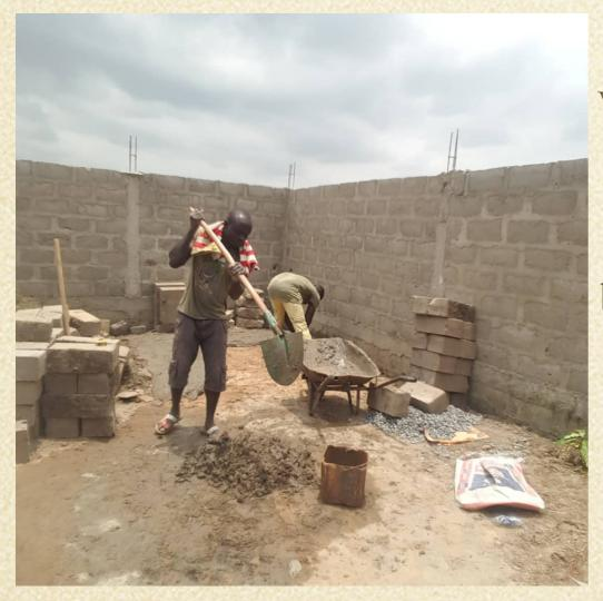
We start by working the sand. Then mix cement with sand and gravel for bricks, planks, and a concrete beam.
