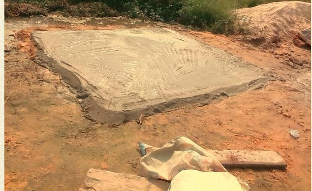
We pour a pad. Then pour the cement planks and the cement beam for the floor and let them dry.
