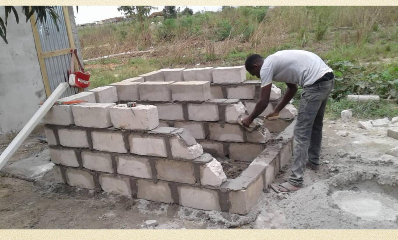
Next, the bricklayer will create the angle for the metal plates that catch the sun and set the notch for the cement beam.
