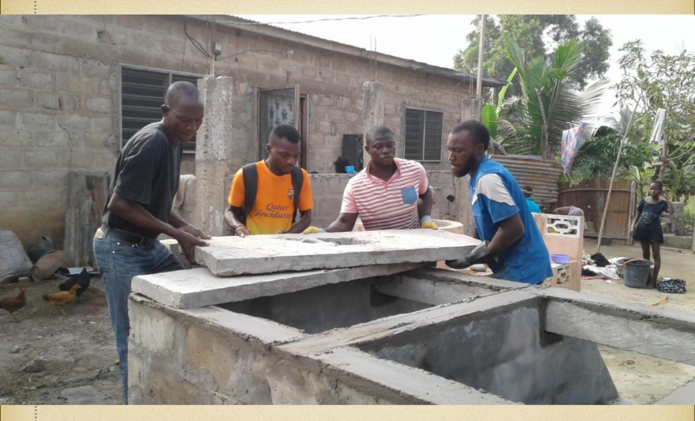
Even with four people, the floor plates are very heavy and must be placed carefully on the wet cement.
